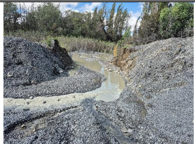
Breach of the stormwater berm along the southern drainage line
