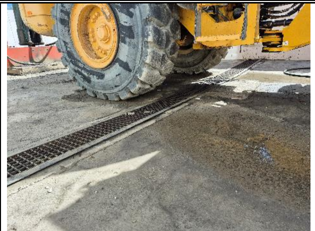
Drain directing waste water of the wash bay to the oil sump
