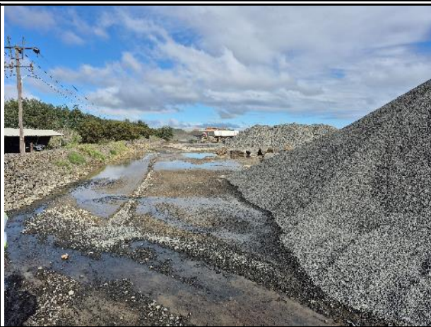
Stockpile area with stormwater berm along the southern boundary
