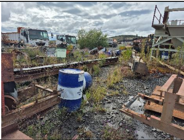
Empty drums to be kept upright and packed in a designated area until removed from site
