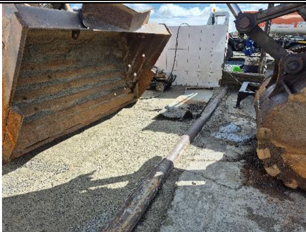
Pipe added to prevent waste water escaping from the wash bay
