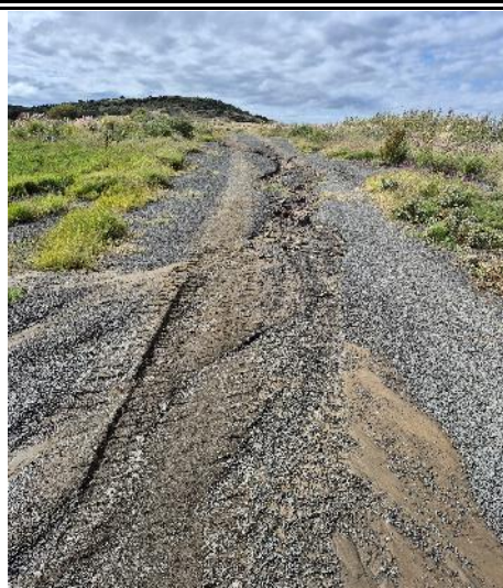
Sheet erosion to be corrected
