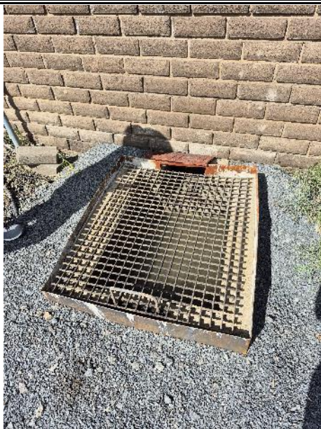
First tank of the oil sump – lid to be considered to prevent infiltration of rainwater
