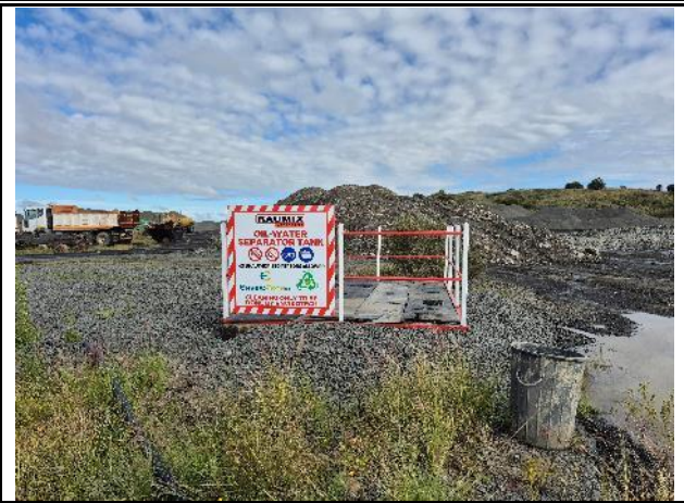
Improved oil sump with clear signage
