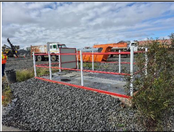
Improved oil sump with clear signage
